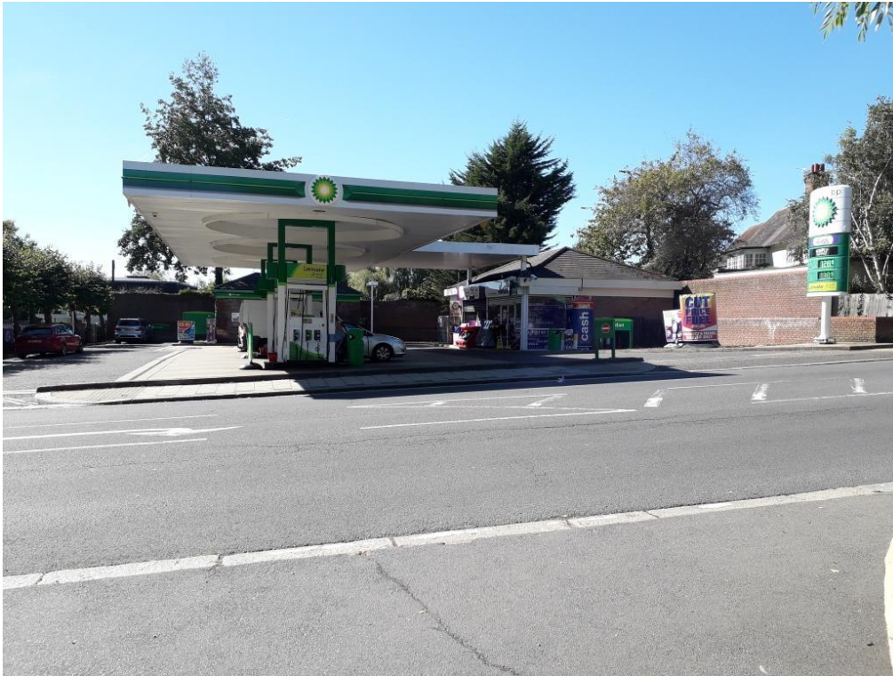
Former petrol filling station
